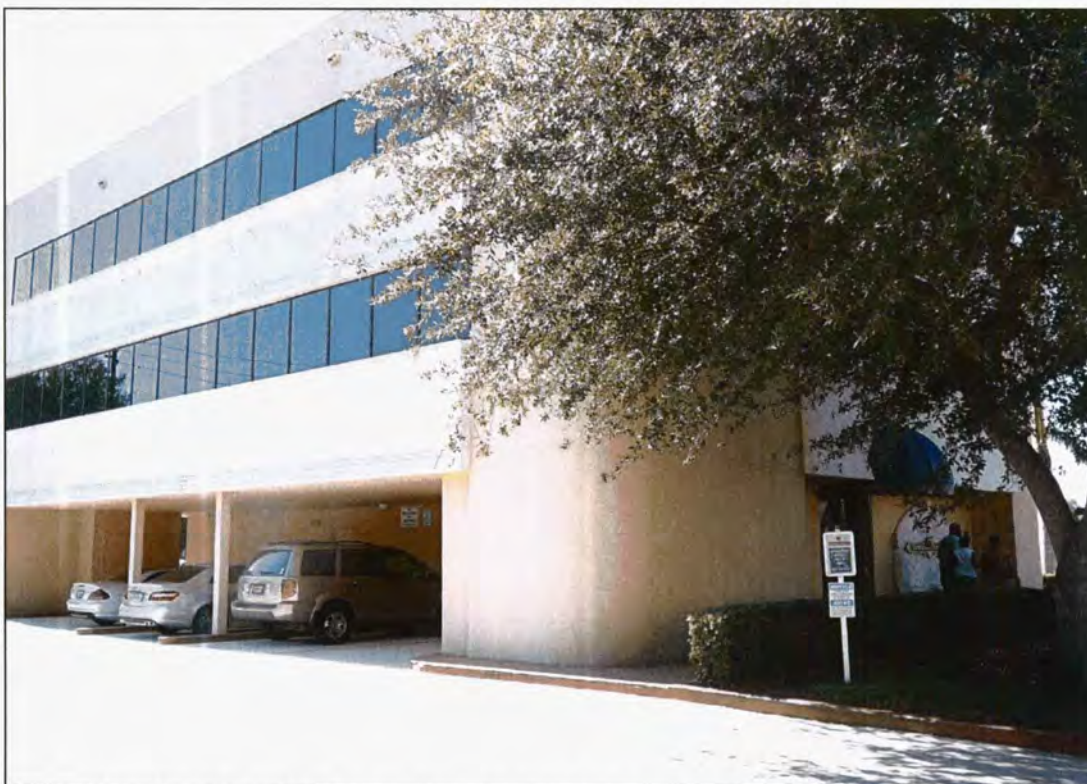
East side - façade includes an awning over the main entranceway.
