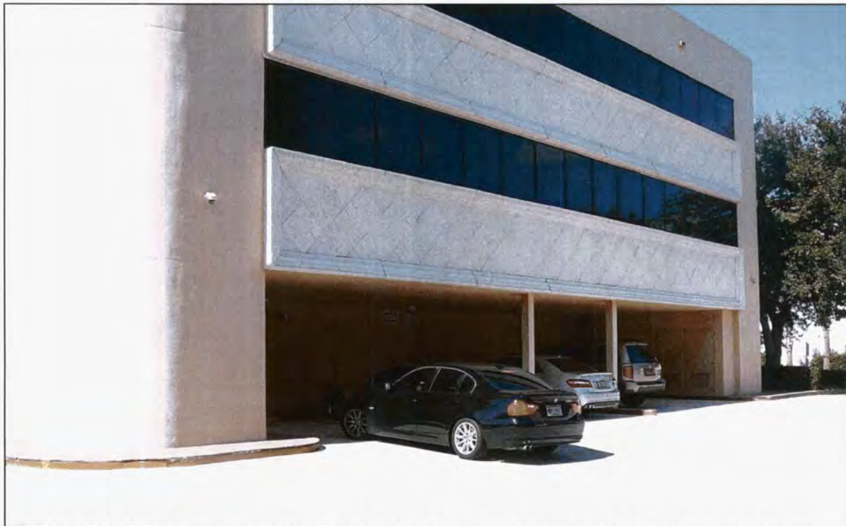
Rear (south) façade – incorporates light-colored pre-cast panels with the diamond design.
