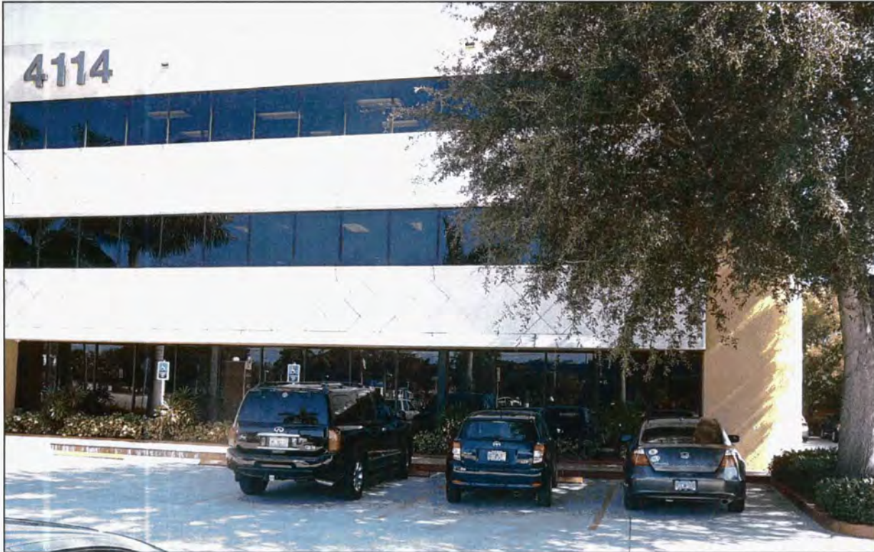
Front (north) façade – incorporates light-colored pre-cast panels with the diamond design and recessed windows.
